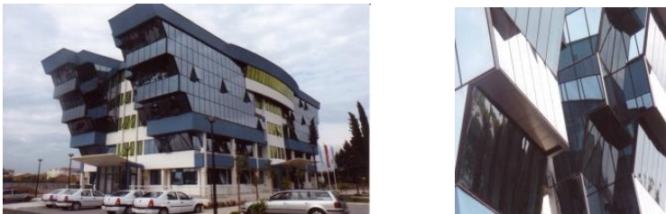
Figure 5 – Semi Structural Solar Facade Serial ALUMIL M3 alutherm
