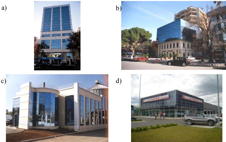
Figure 1 – Some of the construction we have realize
