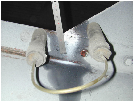
Figure 13 – Inspection of a weld in steel structure
