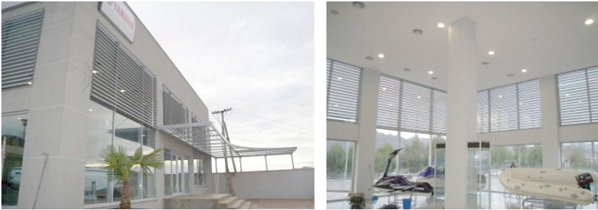
Figure 6 – Building with the natural and artificial light control
